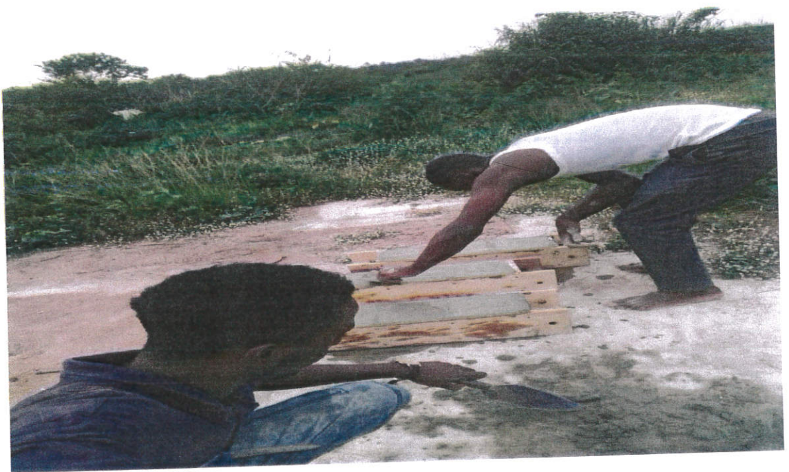
Plate 3.4 Casting of concrete
