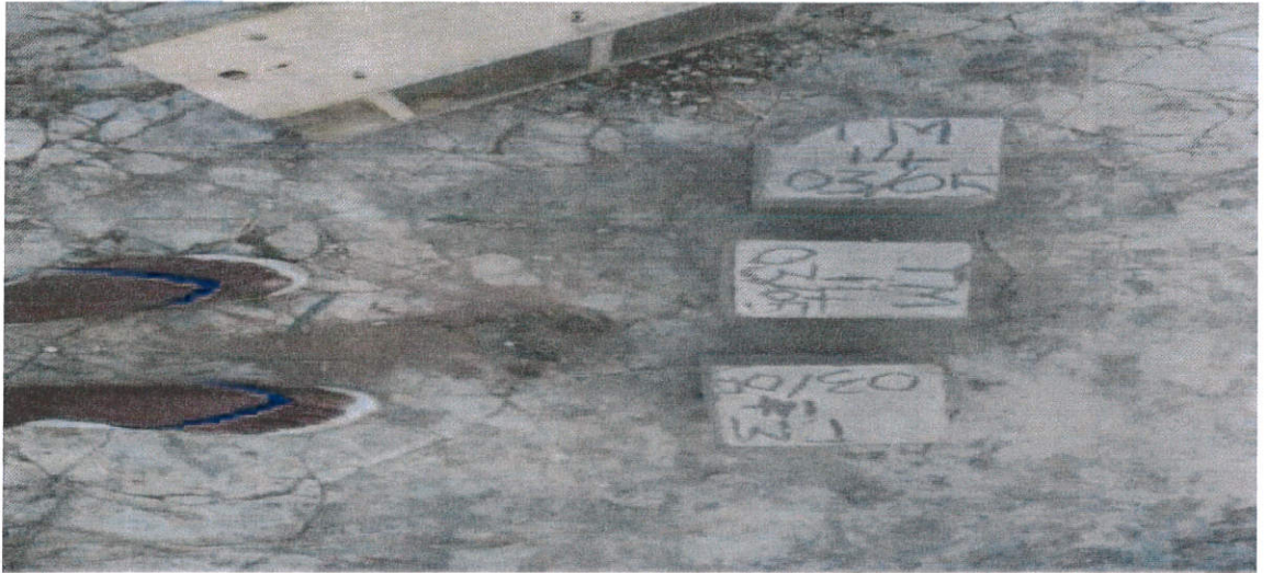
Plate 3.5 Concrete cubes casted
