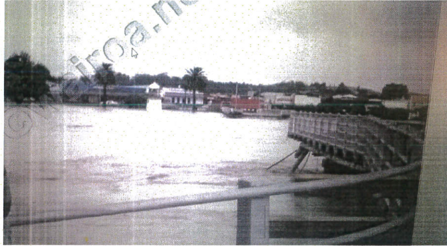
Plate 1.4; the collapsed Wairoa River Bridge, New Zealand, 1988.
