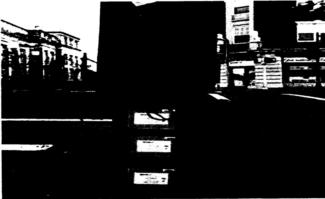
Figure 2.3: Battery backups installed in a separate cabinet from the traffic controller cabinet on the top (Sarah, 2004)
