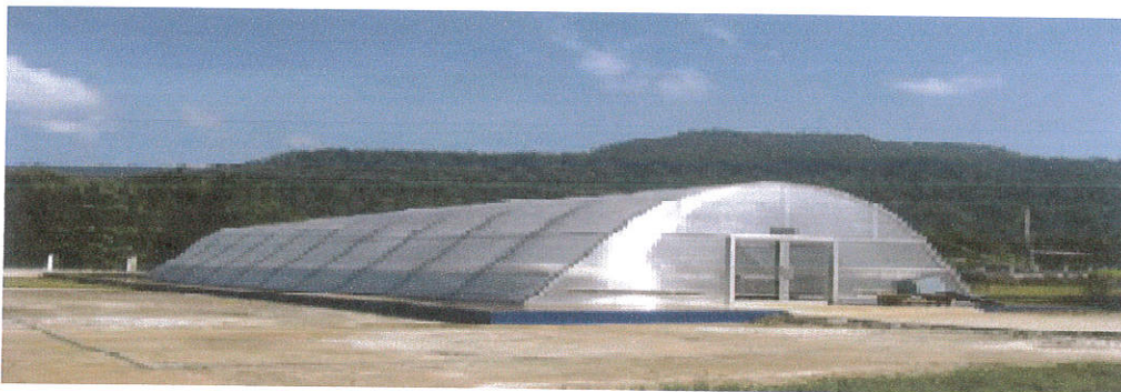
Fig4. A greenhouse solar dryer (Sethi and Arora, 2009)
