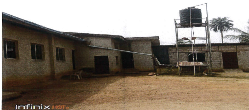
Plate 4.14: Location of rain water harvesting system at Ilotin ACCF.
