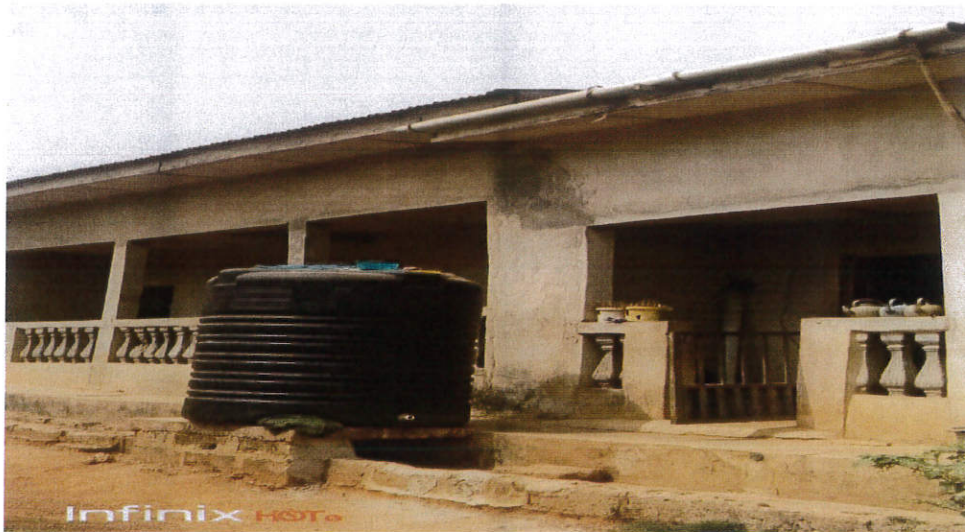
Plate 4.16: Location of Rain water harvesting storage tank at Ootunja.
