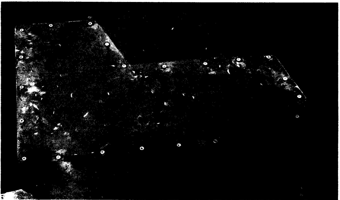
Plate 3.16: The cover plate showing the bolt used for joining the cover plate and the angular bar
