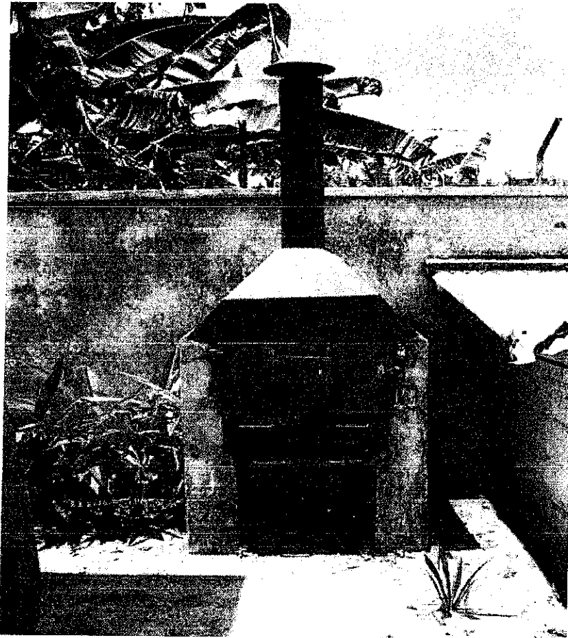
Figure 2 Single chamber incinerator at Ekiti State Waste Management Board
