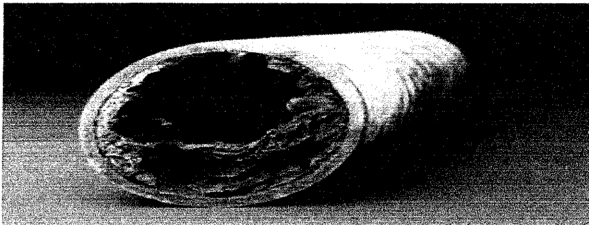
Figure 2.8: Pipeline affected by Microbial Induced Corrosion (MIC)
