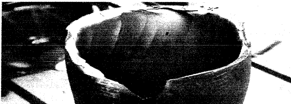
Figure 2.6: Oil and Gas Pipeline after being attacked by Stress Corrosion Cracking.
