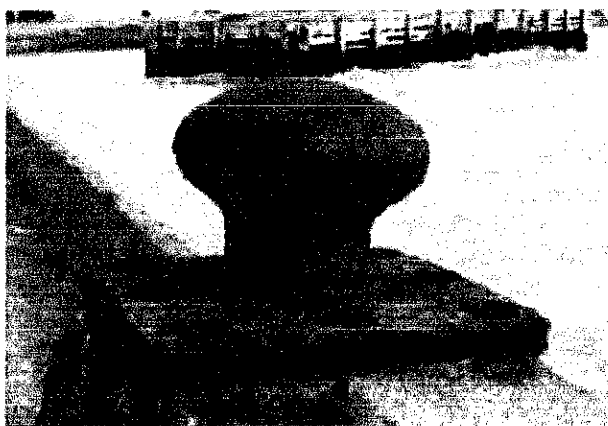
Figure 2.2: Uniform Corrosion
