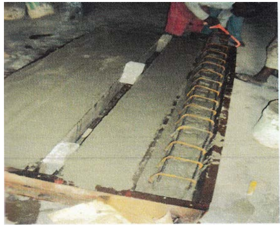
Figure 4: Foamed aerated concrete beams concreting operation
