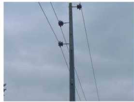
Fig 5. 11KV line without a broken cross arm.
